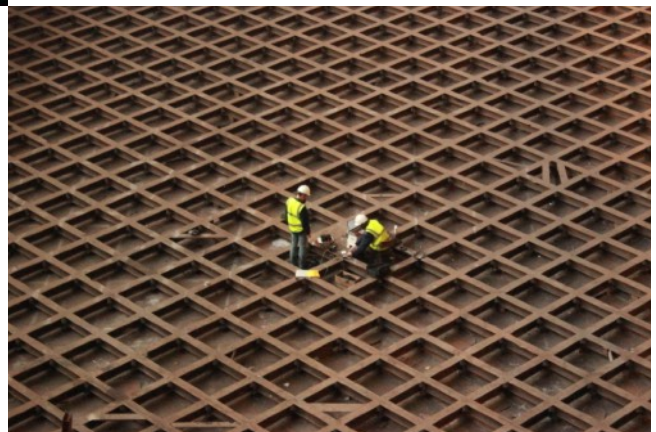
FERA_ID EXCAVATION SITE #2: SHIPYARD LANDSKRONA, SWEDEN, 2016
